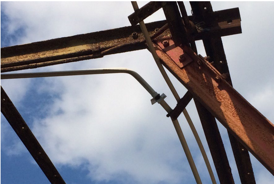
Rail tracks recycled at the 1930's sheds- Haifa East Station - photo by Ruth 2018.
